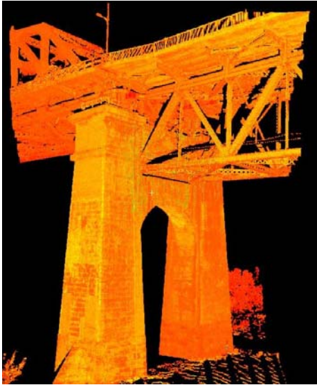
Figure 1: 3D laser scan of Jacques Cartier Bridge tie-down pier
